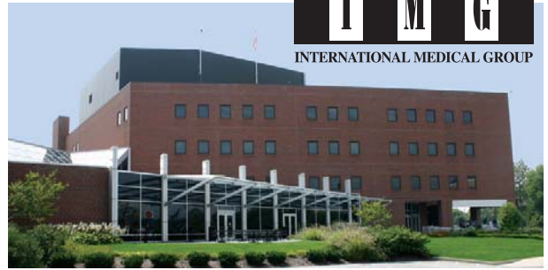
IMG World Headquarters, Indianapolis, Indiana
